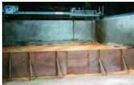
NEW 2000 TONNE STORE WITH 3.65 METRE STORAGE AND TEMPERATURE DRYING SYSTEM
